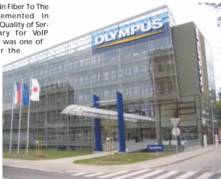
The new Olympus branch in Prague
