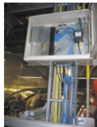
MICROSENS switches along the welding line
