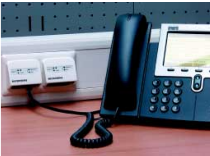
IP-Telephony with the new MICROSENS switches.
