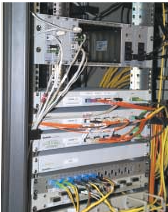
The used hardware (from top to bottom): modular SM/MM converter systems (3HU), 3x CWDM multiplexer with a redundant power supply unit (RPSU)
